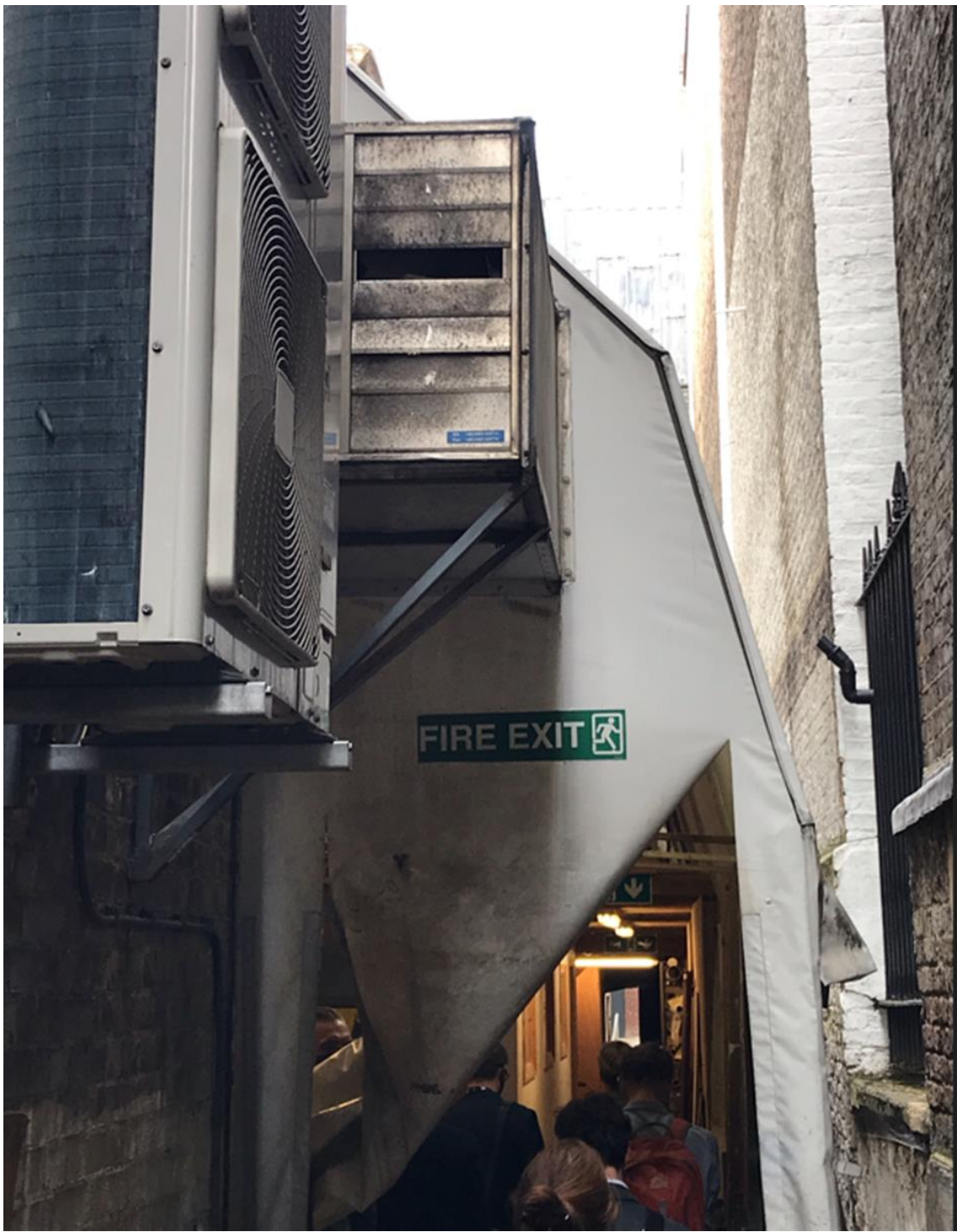
View of East Yard looking north. Albany on the right.
